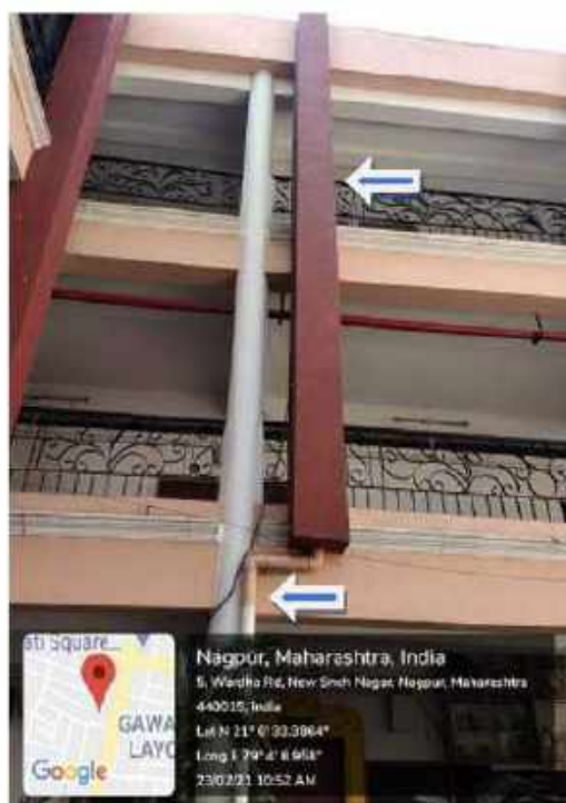
Pipeline of Water Harvesting System
