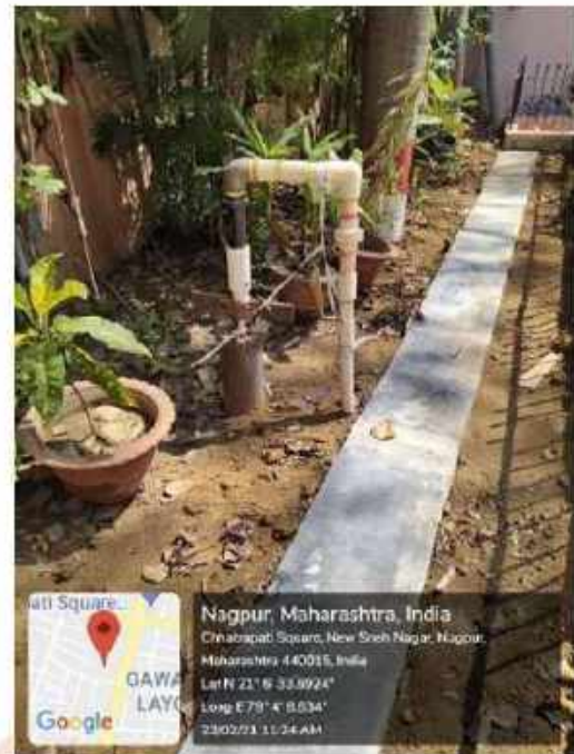
Bore well in college
