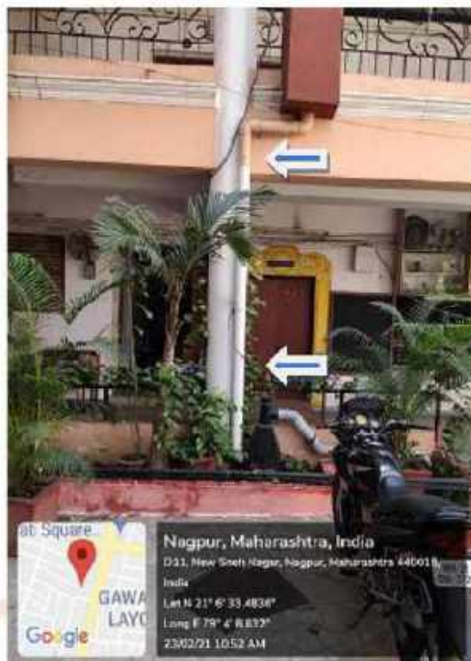
Pipeline of Water Harvesting System
