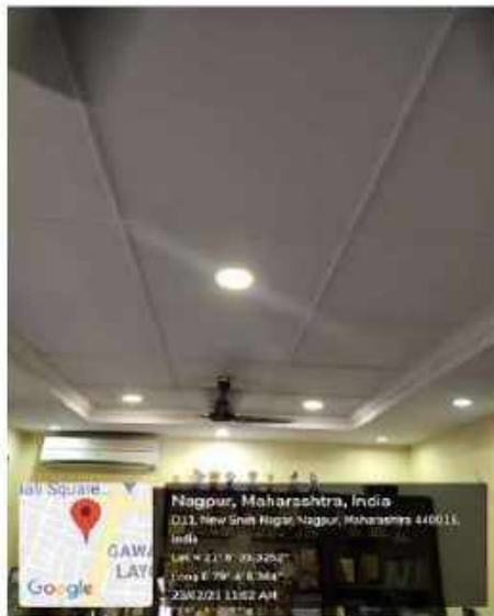
Use of false ceiling to reduce air-conditioned volume and reducing AC load
