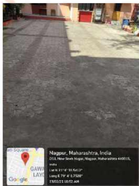
Catchment Area for Water Harvesting
