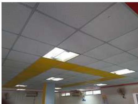
False Ceiling at computer laboratory
