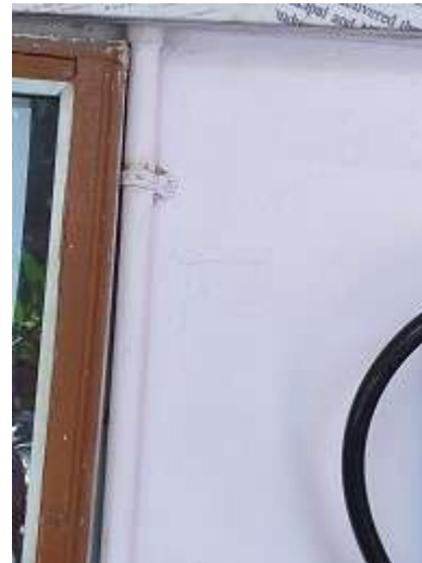
Pipeline used to supply AC Condensed water to trees
