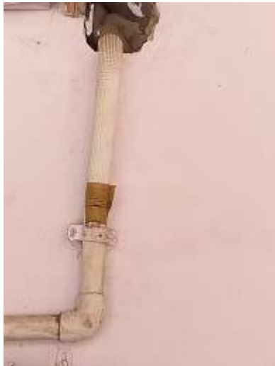
AC Condensed Water used for gardening
