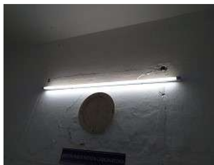
FL Tube Lights Replaced By LED Tube Lights
