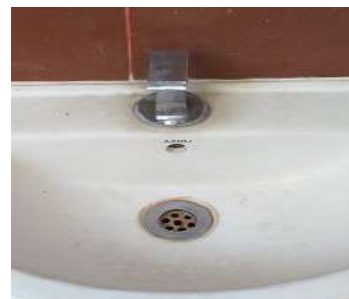
New taps installed in toilets
