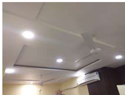
FL Tube Lights Replaced By LED Lights
